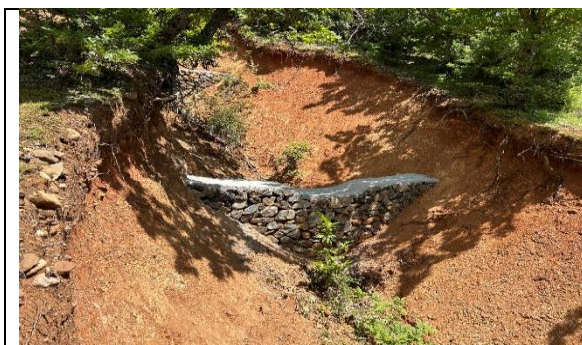
Figure 7 - Buid stone check dams in Korthpulë
